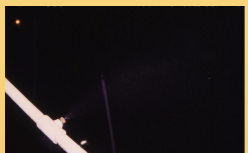
Misting adds water to the air to compensate for losses. Although not an ideal approach, misting provides protection while issues are addressed.
