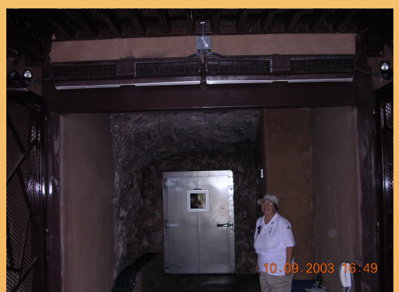
An air curtain was added to assist with climate and lint control.
