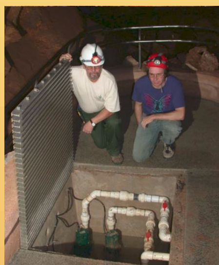
Trails with integrated curbing and tread allow washing to remove dirt and lint. Sumps collect the wash water for removal from the cave.
